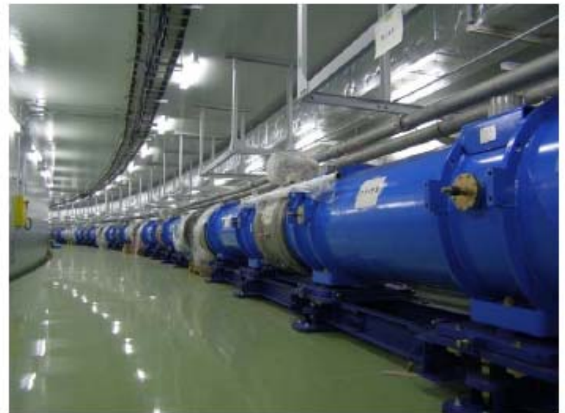
Superconducting magnets for the neutrino beamline
