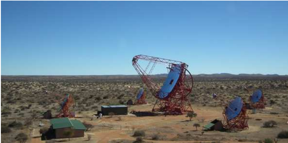
Figure 2.56: The H.E.S.S. IACT array in Namibia, showing the four 12-metre telescopes of HESS-I and the new 28-metre HESS-II. Photograph from [245]
